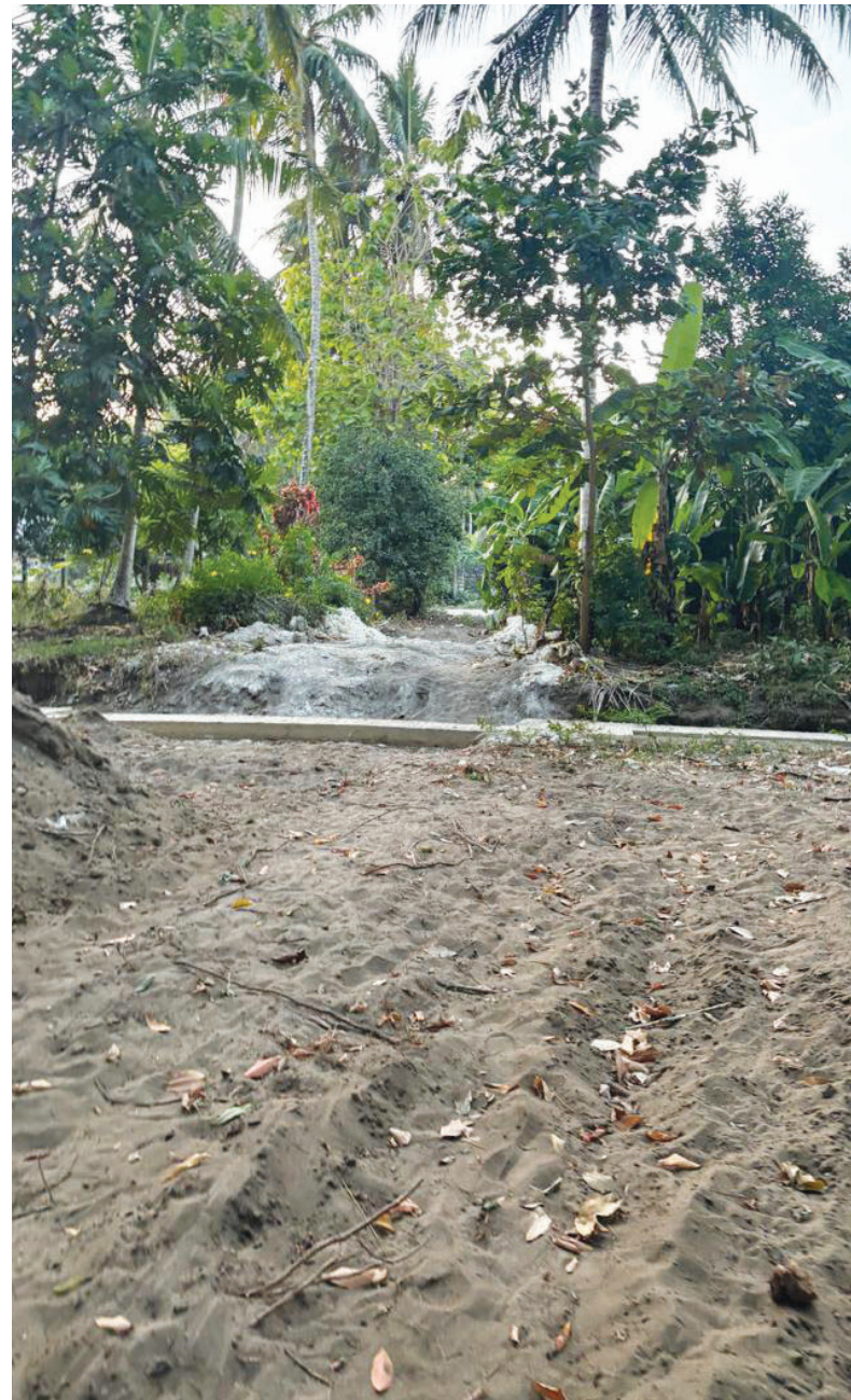
Construction of the hotel going on. Photo: Our Photographer
